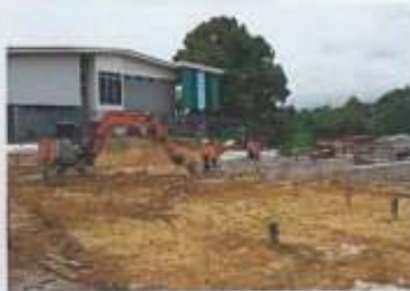
SSC Honiara landing station construction
